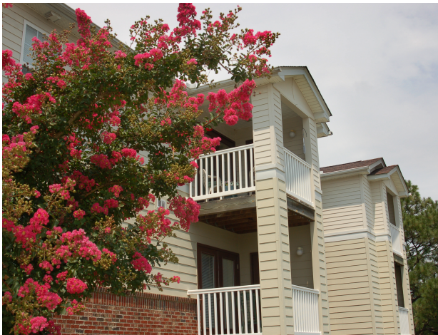
FERNWOOD HALL APARTMENTS, LEXINGTON COUNTY
