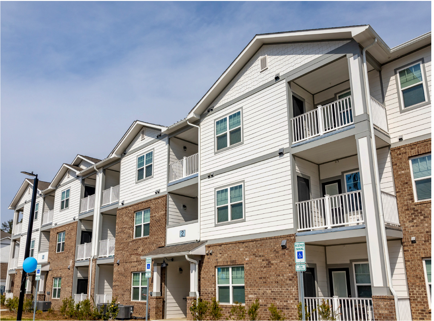
The Village at Congaree Pointe in Columbia opened in early 2024 and provides 240 affordable units.
