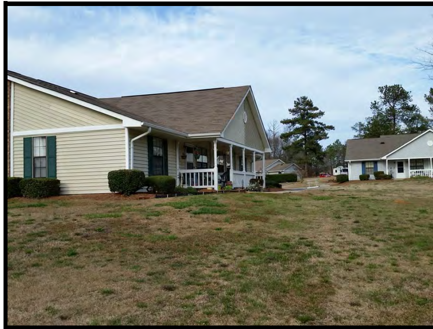
View of site from the southwest
