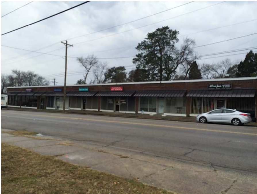
Looking West From Site (Southern End)
