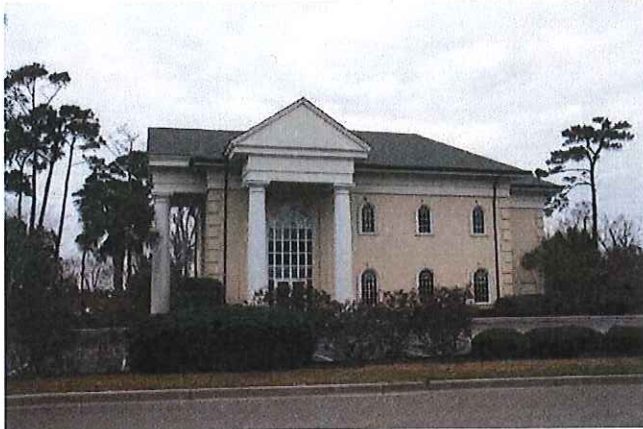
TD Bank adjacent to west of site Facing west from Oleander Drive
