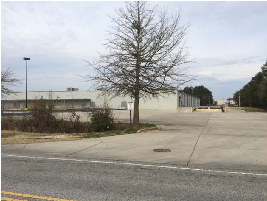
Looking southwest from site
