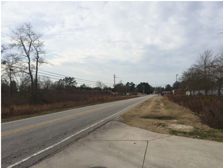
Looking southwest on Wise Drive
