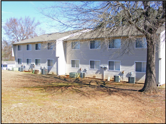
Typical units - rear view
