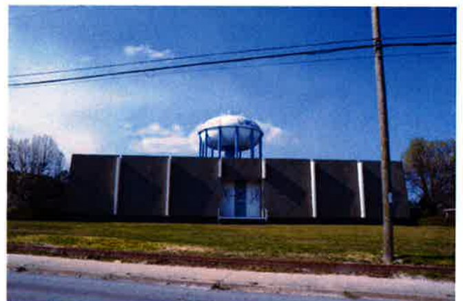
Adjacent AT&T facility and City water tank located along Horseshoe Circle to the southeast and east of the Site.
