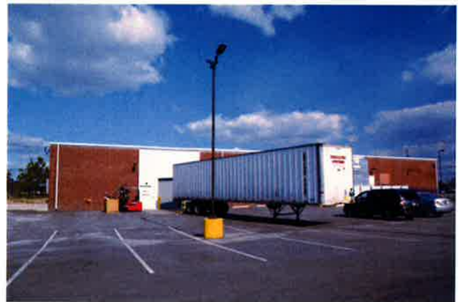
Adjacent Harbor Freight Tools located to the southeast of the Site.
