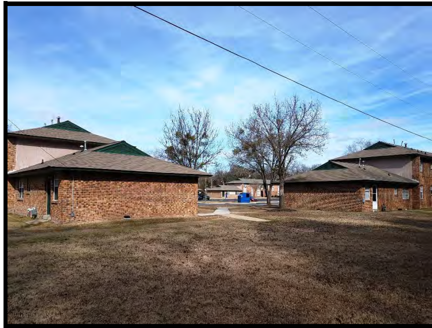
View of site from the southwest
