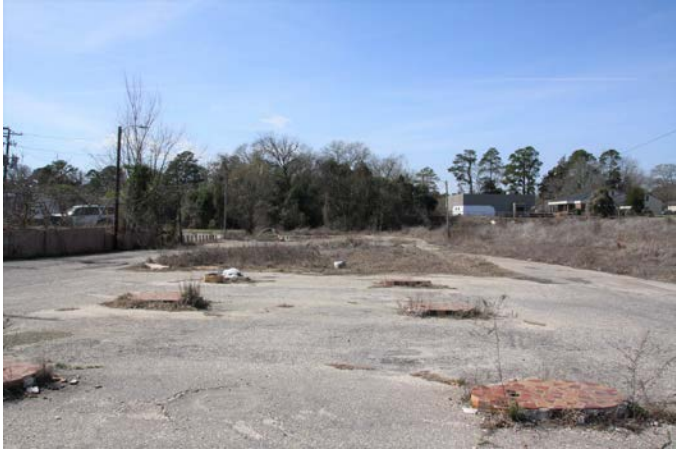
SITE – The Belmont Apartments 719 S. Irby Street, Florence, SC Facing west from Irby Street
