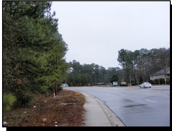
View north on O'Neil Ct., at site
