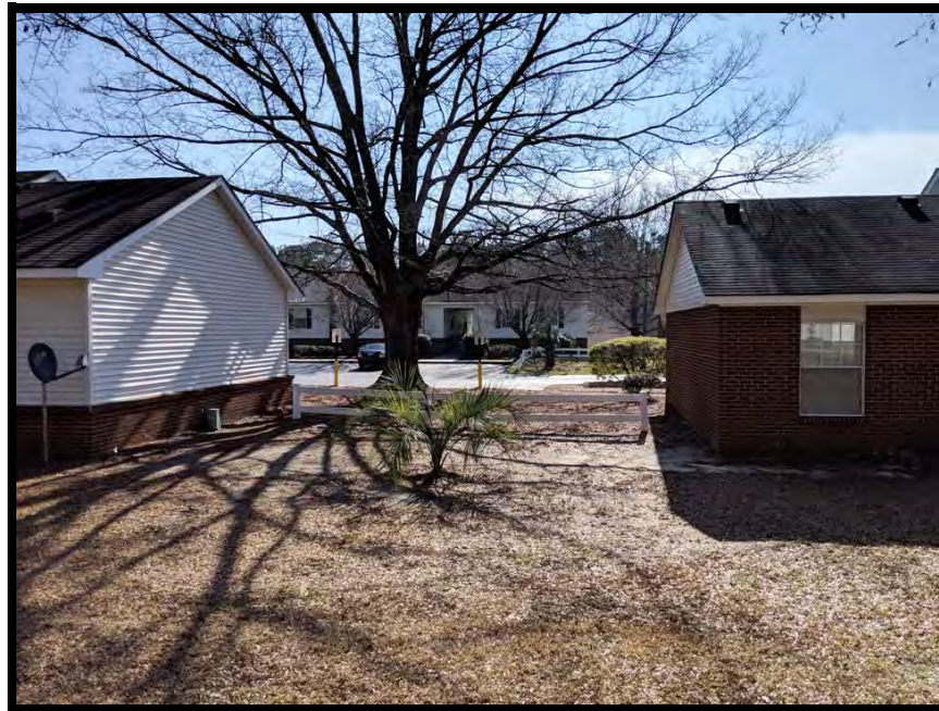
View of site from the north
