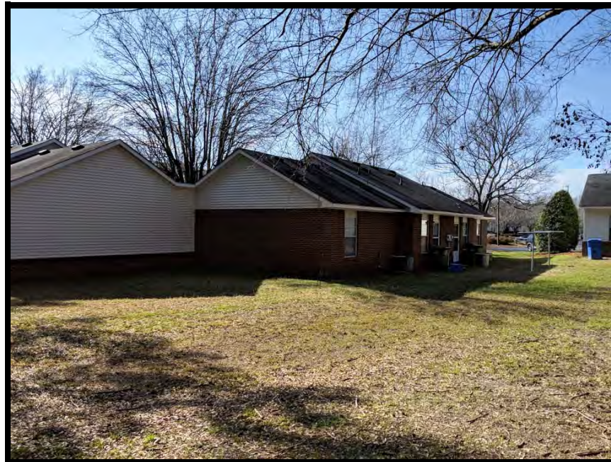
View of site from the northeast
