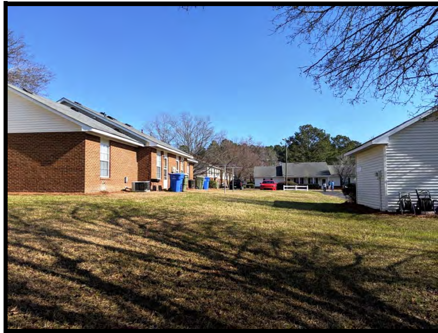
View of site from the west
