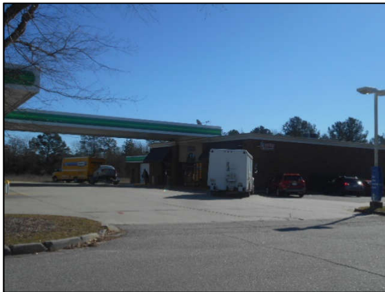
A BP service station just northwest of the site
