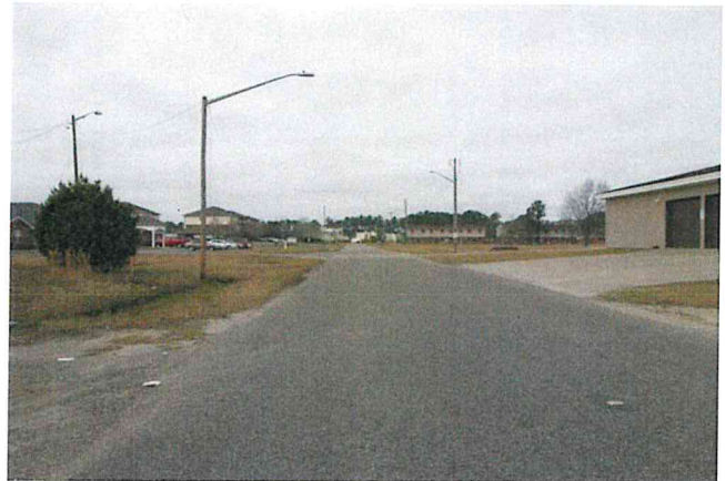
Facing west along Lincoln Street Site is on left Georgetown Housing Authority is on right
