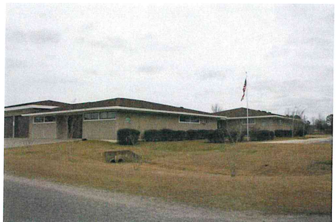
NORTH – Georgetown PHA Community Building Adjacent to north of site Facing north from Lincoln Street
