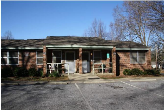
Multi-family apartments adjacent to west of site Spartanburg Housing Authority
