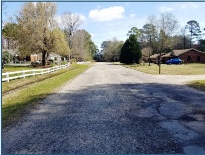
Streetscape: Northeast view of Richmond Street
