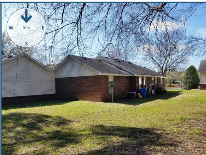
View of site from the north
