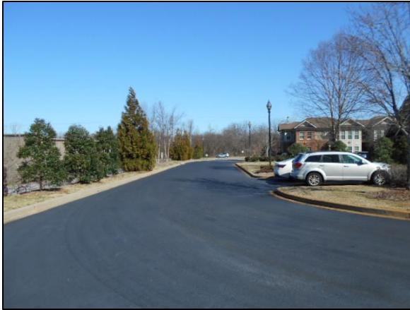
Existing entrance road facing north.
