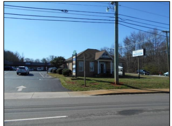
Commercial building to the north.
