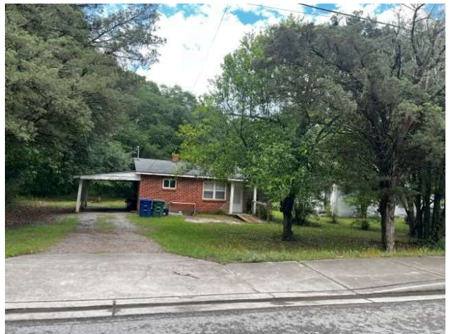
Single-family home west of Subject site
