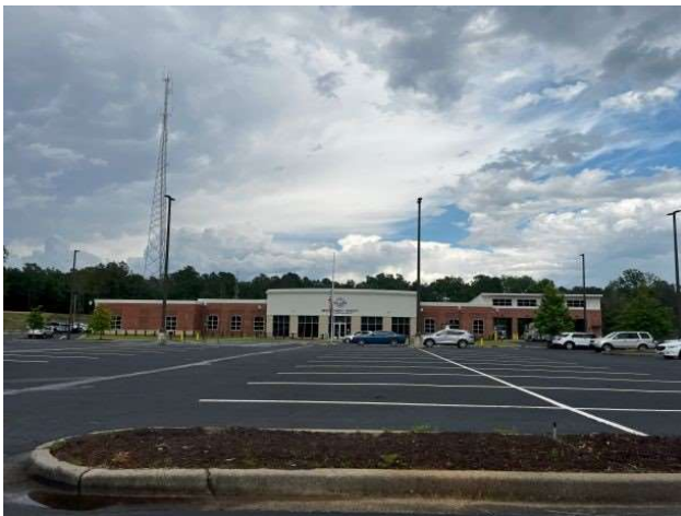
Government building east of Subject site
