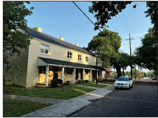
Existing building along Nassau Street
