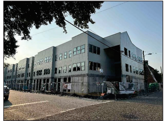
Archer School Apartments (under construction) to the south
