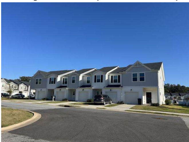
Farrs Bridge Towns to the east of Subject
