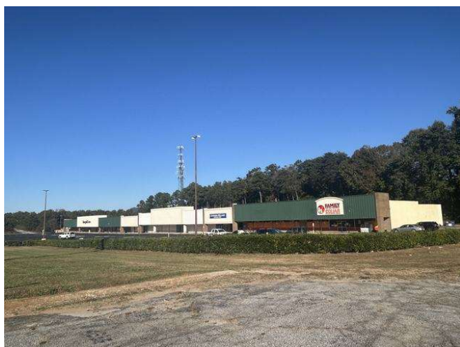
Retail use along White Horse Road to the north of Subject
