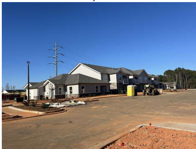
Adjacent Cherokee Landing Phase I under construction
