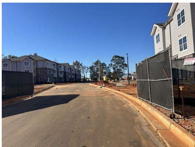
Adjacent Cherokee Landing Phase I under construction
