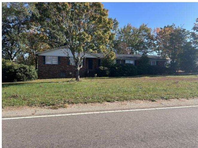
Single-family home across Berea Heights Road from Subject
