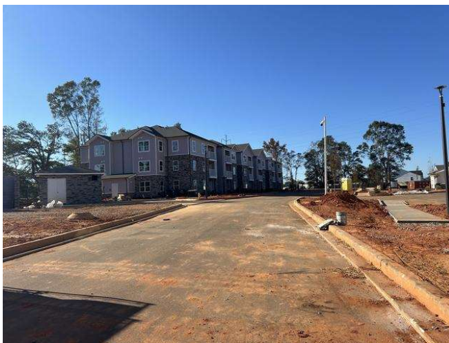
Adjacent Cherokee Landing Phase I under construction
