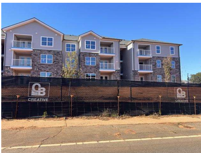
Adjacent Cherokee Landing Phase I under construction
