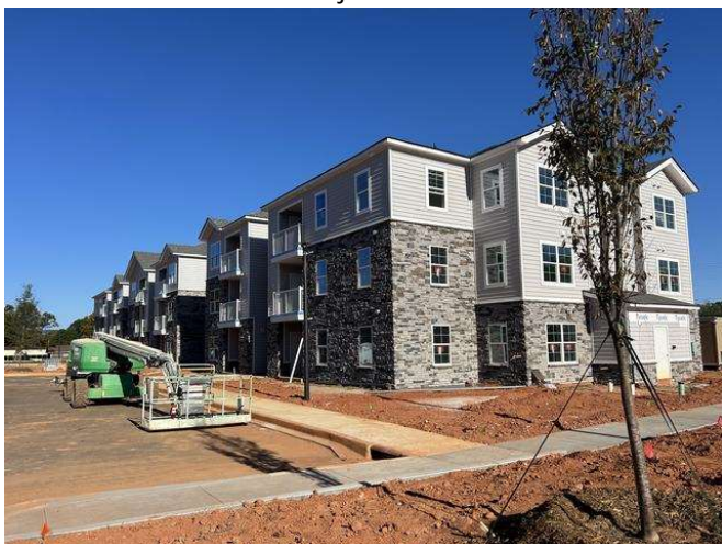
Adjacent Cherokee Landing Phase I under construction
