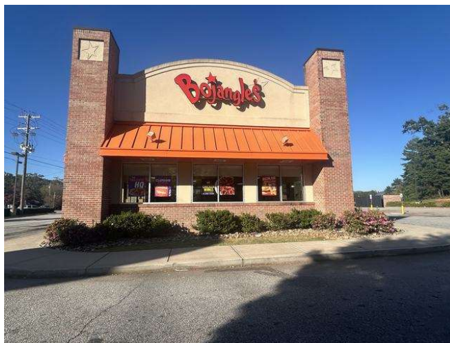
Retail use along White Horse Road to the north of Subject
