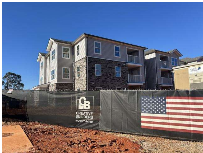
Adjacent Cherokee Landing Phase I under construction
