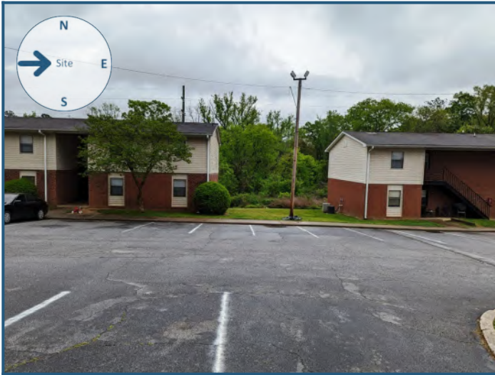
View of site from the west
