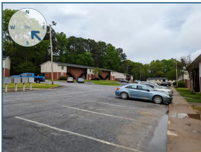
View of site from the southeast
