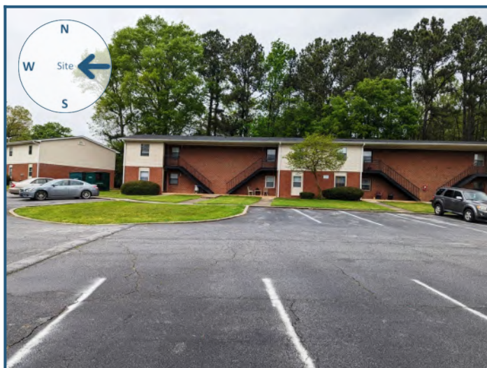
View of site from the east
