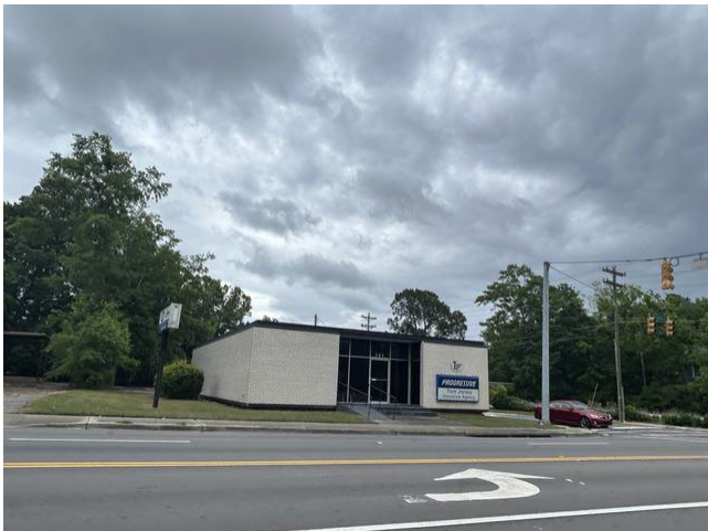
Commercial use east of Subject site
