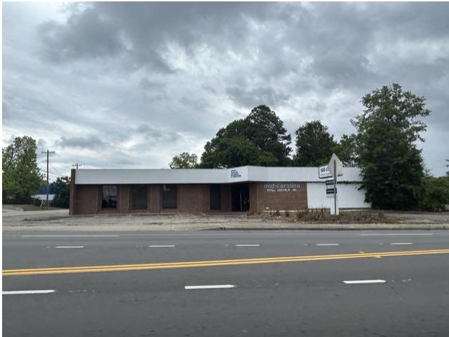
Commercial use east of Subject site
