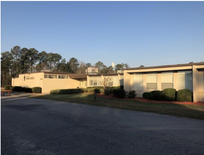
View of Navigation Driving Academy abutting to the south
