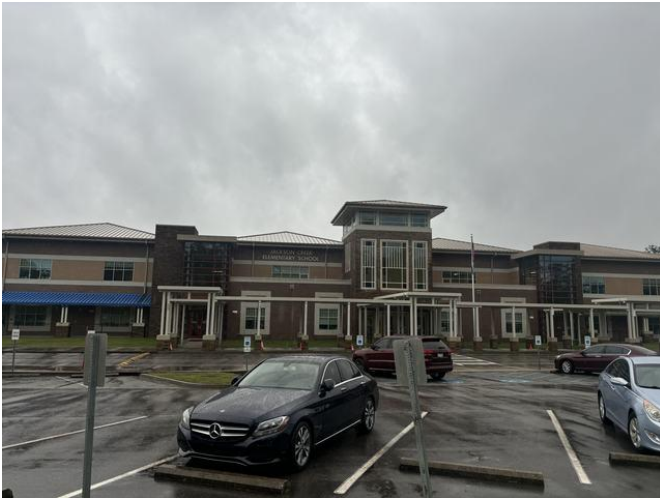
Jackson Creek Elementary southeast of Subject site
