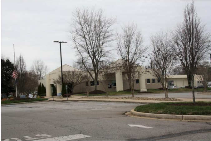
WEST – Utility company adjacent to west of site Facing west from parking lot near edge of site Site is to the right of building
