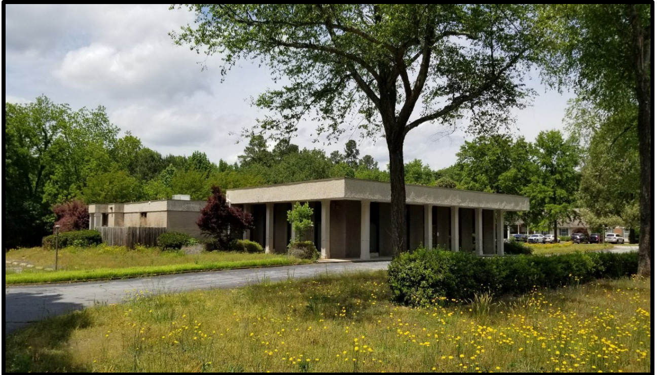
Photo 13 – nearby vacant office building
