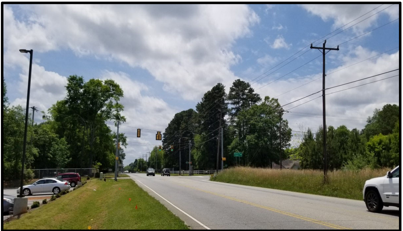
Photo 4 – looking south on Cannons Campground Road
