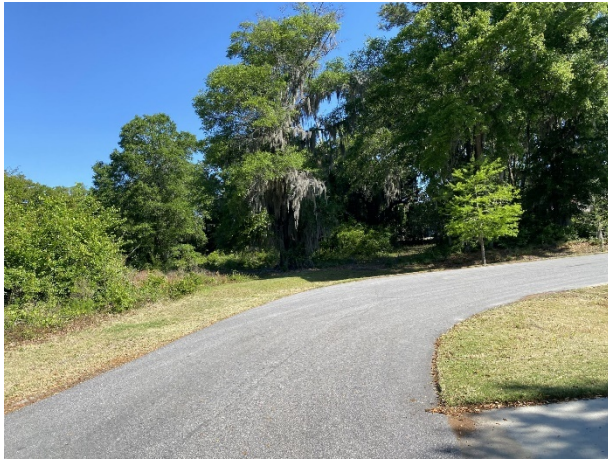
View north along Bowling Lane
