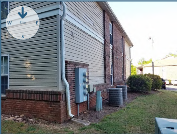
View of site from the north
