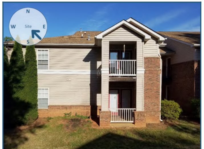
View of site from the southeast
