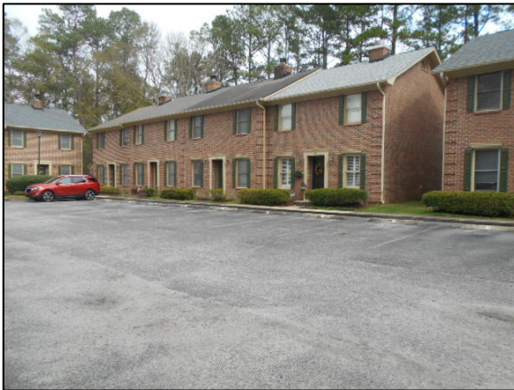
Coventry Place Condominiums west of site.
