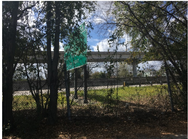
View west of Subject site
