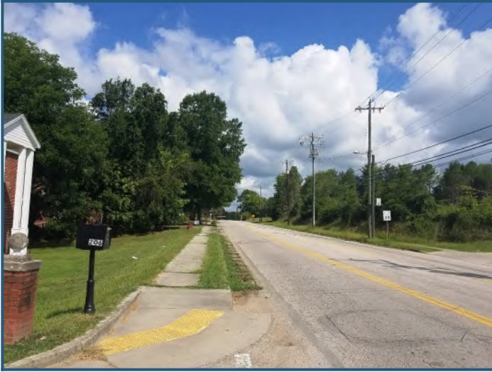
Streetscape: Northwest view of Center Street
