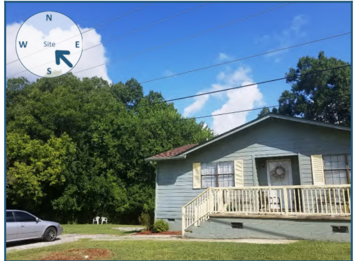
View of site from the southeast
