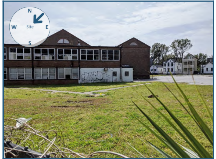
View of site from the northeast
