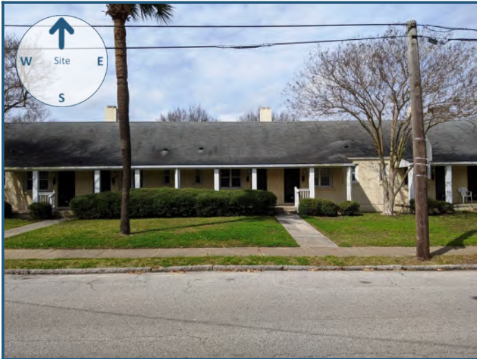
North view from site
