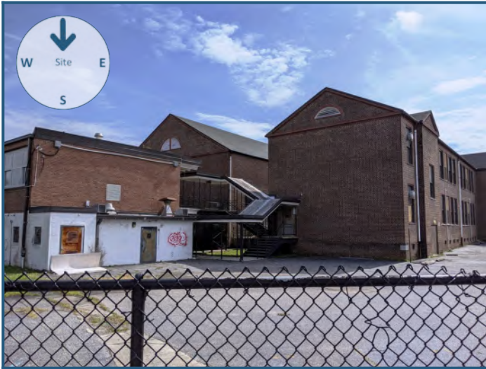
View of site from the north
