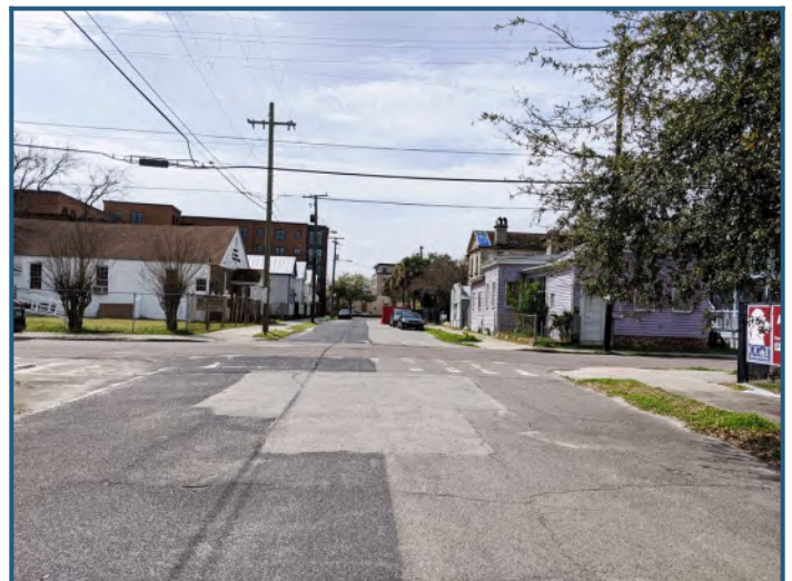
Streetscape: West view of Jackson Street
