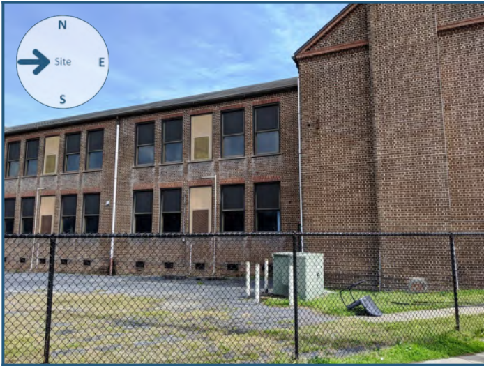
View of site from the west
