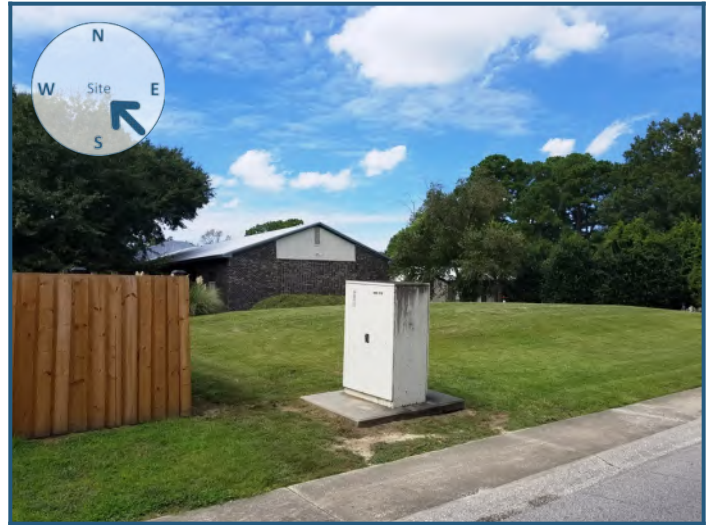
View of site from the southeast
