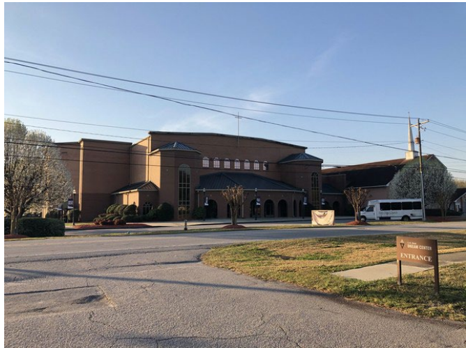
View of church located across Atlas Road
