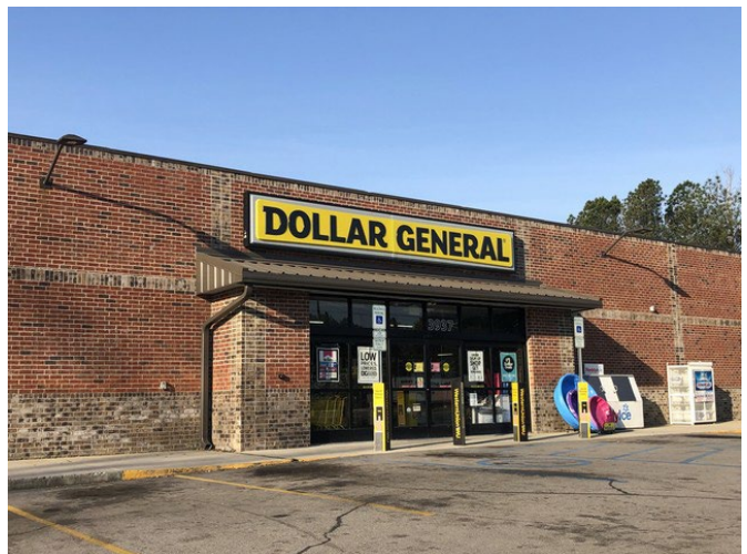
View of Dollar General to the west
