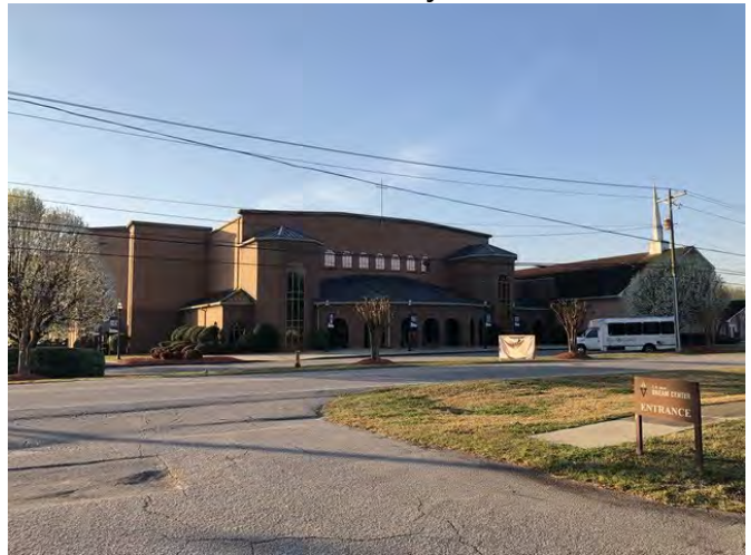
View of church located across Atlas Road
