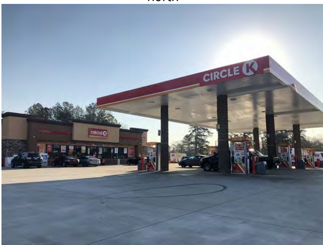
View of gas station/convenience store to the west
