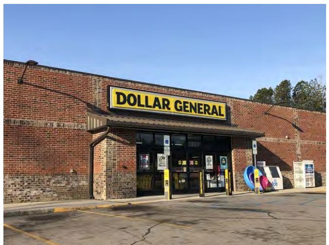
View of Dollar General to the west
