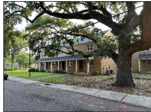
Existing building on east side of Nassau Street
