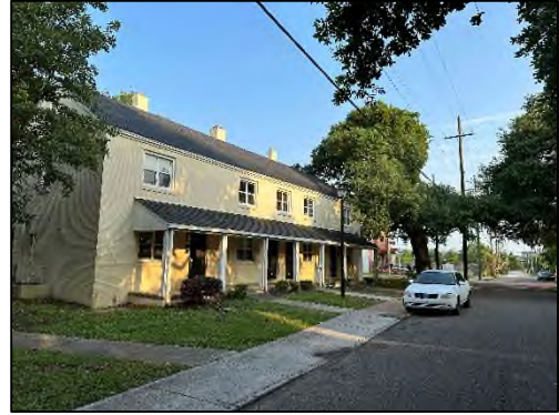
Existing building along Nassau Street
