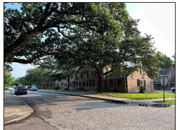
Meeting Street Manor Apartments to the east
