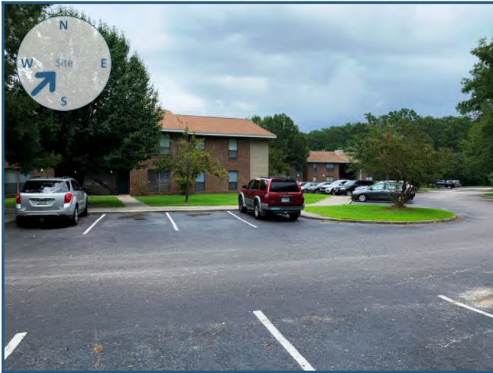
View of site from the southwest
