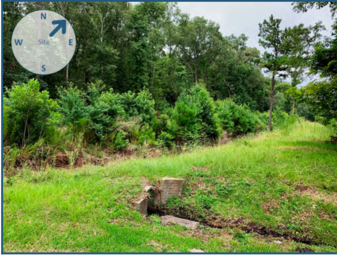
Northeast view from site
